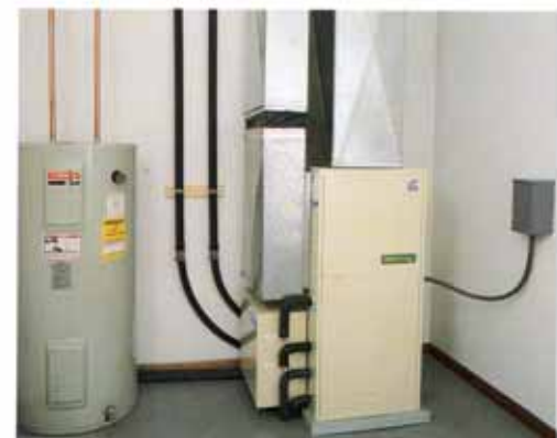
A GeoSource heat pump is easy to install. Its PumpPAK™ incorporates all pumps and valves into one unit.
